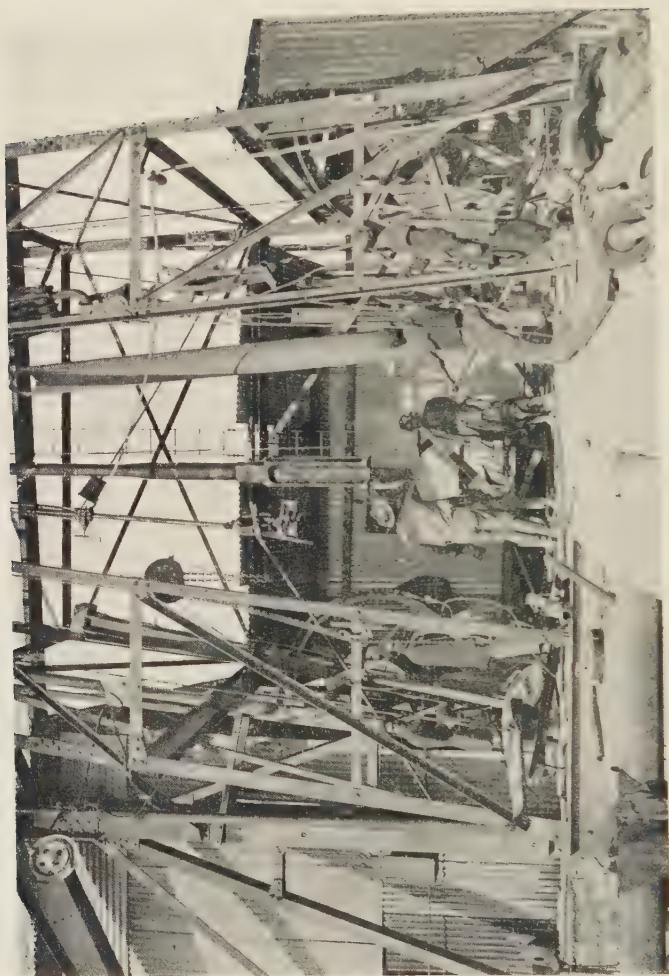
THE DERRICK FLOOR OF A STANDARD TYPE DRILLING RIG, SHOWING THE HEAVY CABLE BIT WHICH POUNDS ITS WAY THROUGH THE ROCK
