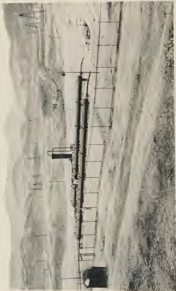
GAS SEPARATORS FOR SEPARATING THE GAS FROM THE OIL AS IT FLOWS FROM THE WELL IN THE OIL FIELD ON THE MAIDAN
