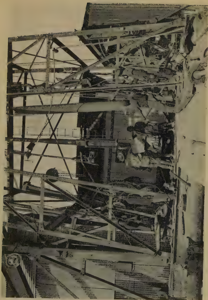
THE DERRICK FLOOR OF A STANDARD TYPE DRILLING RIG, SHOWING THE HEAVY CABLE BIT WHICH POUNDS ITS WAY THROUGH THE ROCK
