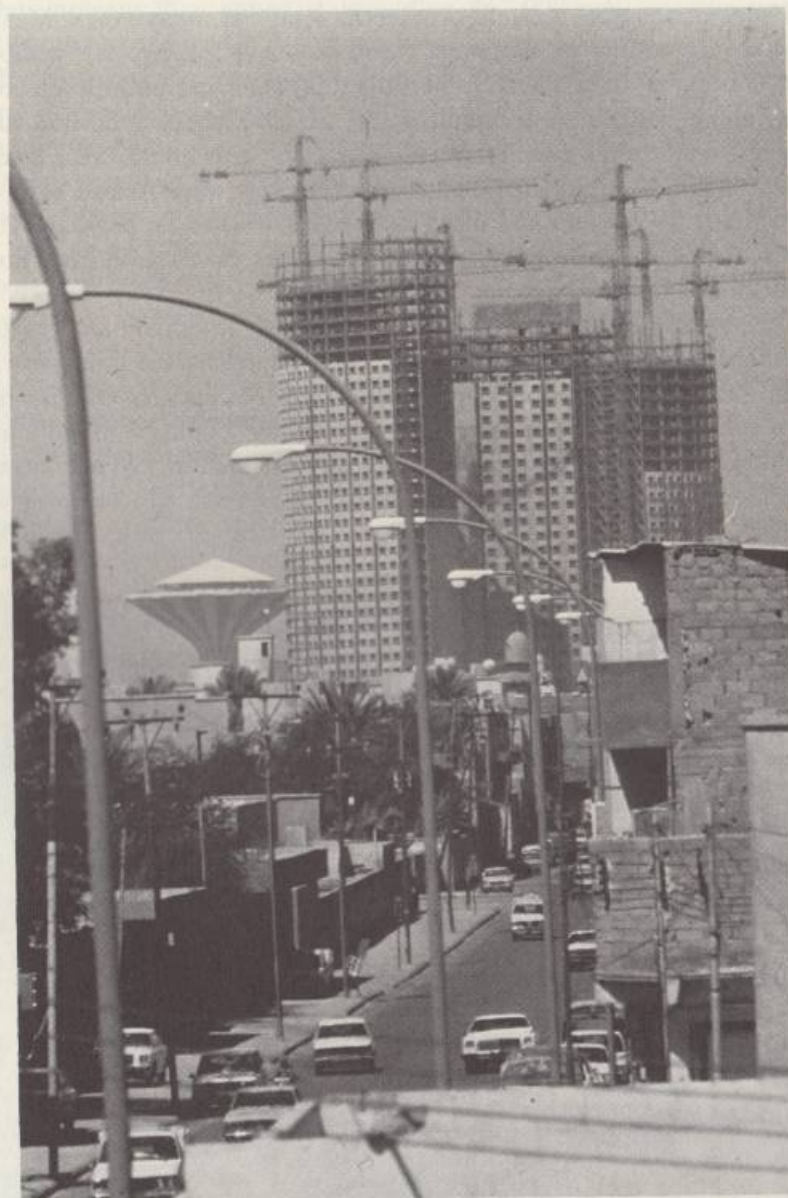
Riyadh buildings under construction, 1980 (courtesy of Aramco World Magazine. Photographed by S. M. Amin)
