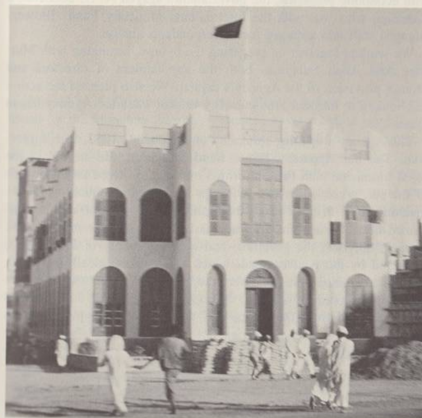
The Saudi Arabian Monetary Agency, original Jidda building before and after remodeling, 1952 (taken by the author)
