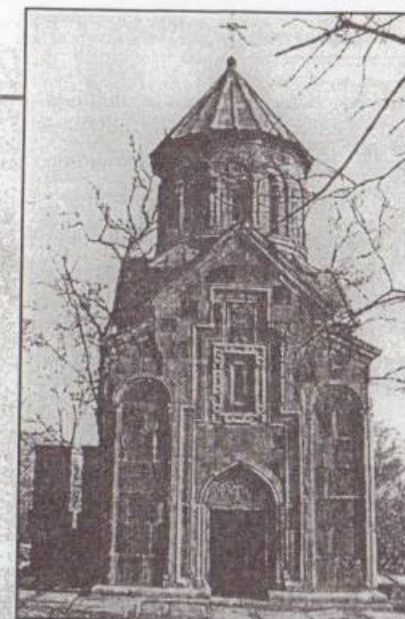
Kotayk marz, Garni, church St. Astvatsatsin, (XIV c.). Project director – Gagik Soghomonyan, head of the construction – Samvel Stepanyan (reconstructed in 1984-1989).
