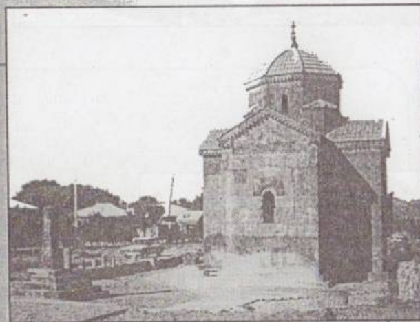
Aragatsotn marz, Talin, church St. Astvatsatsin (VII c.). Project director – Mery Danielyan, head of the construction – Grigor Vardanyan, sponsor - Andranik Daglyan (reconstructed in 1998).
