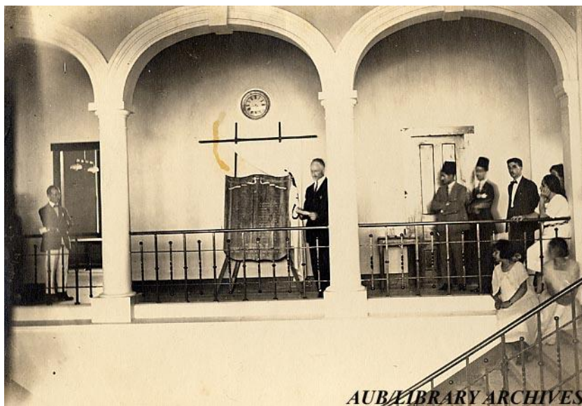
Memorial tablet erected at West Hall and dedicated to the memory of 32 SPC medical alumni who died while on active service in the Ottoman Army during WWI. (Source: AUB Archives)
