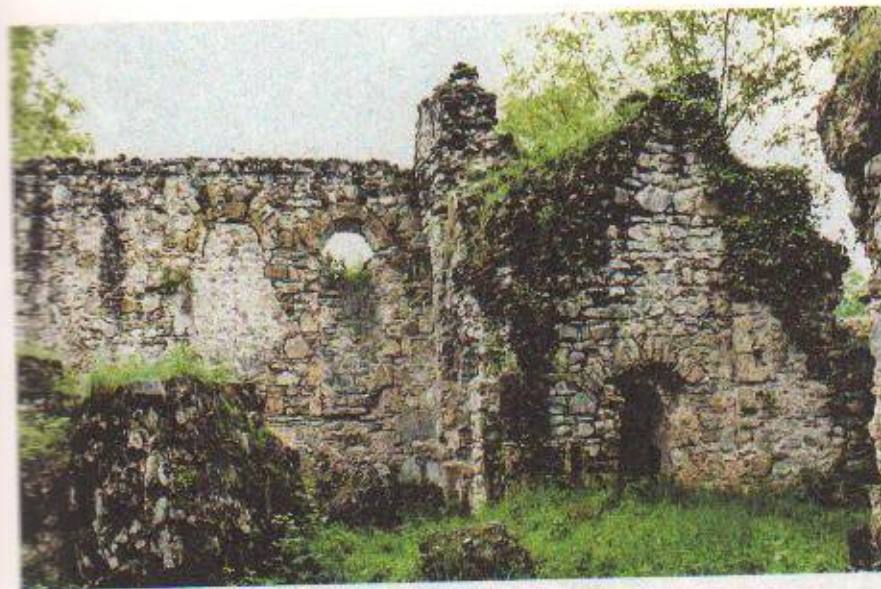
Fig. 8: Yeddi Kilsa. Western church. North wall and northeast sacristy seen from the south.
