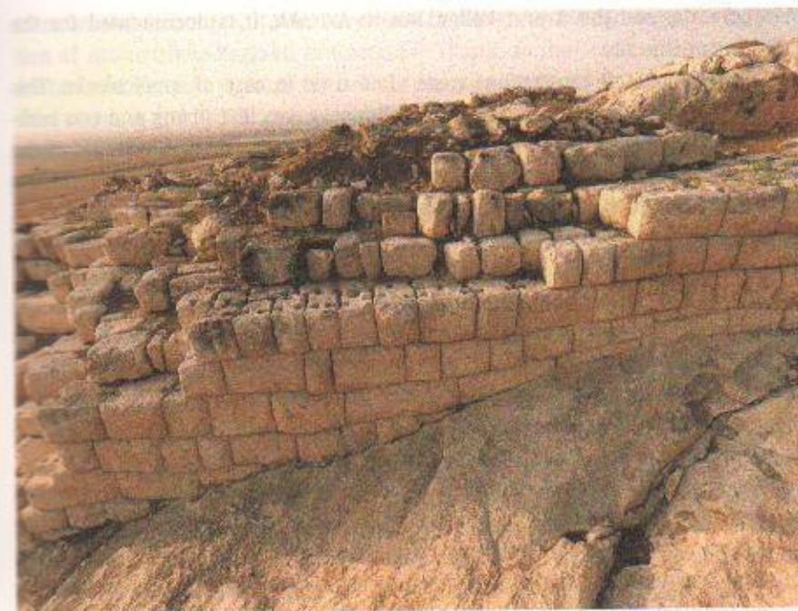
Fig. 7: Horizontal polished surfaces of the quadras, rustic elaboration of the outer faces, facets and "swallow-tail" connections of the northern fortification wall, 2009.
