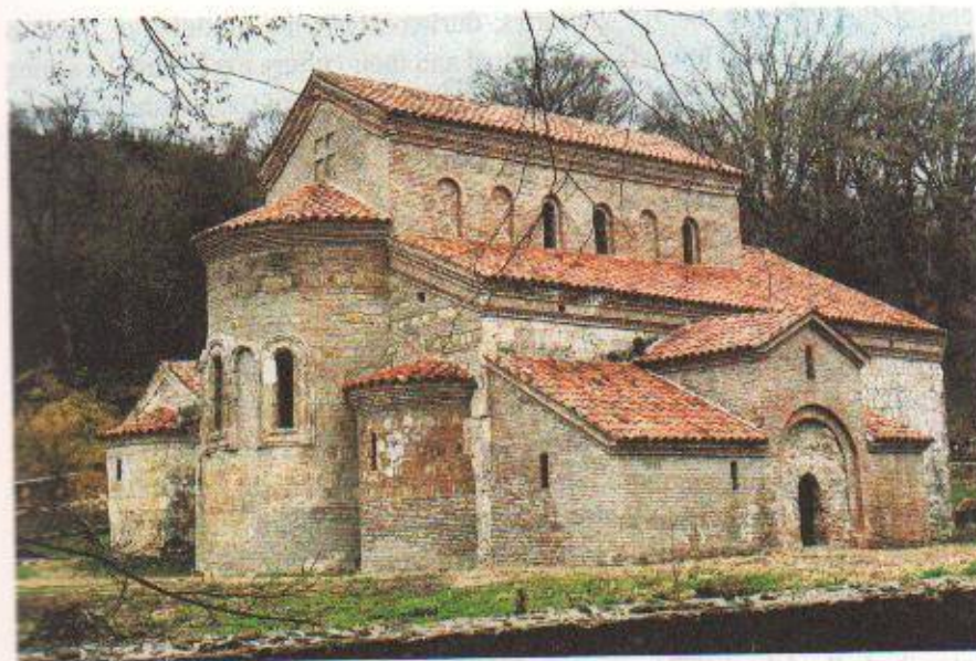
Fig. 13: Vazisubani, Kakheti (Georgia). Sanagire. General view from northeast.
