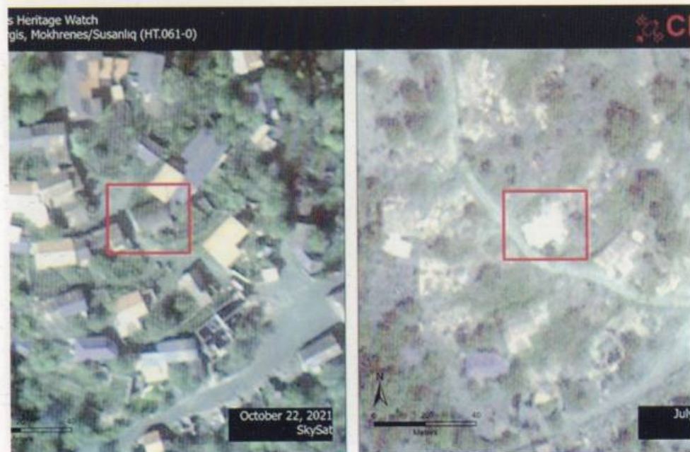
17b. Complete Destruction of St. Sargis Church After the Occupation by Azerbaijan
